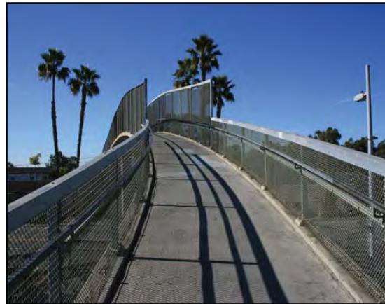
Pedestrian bridge over I-5
