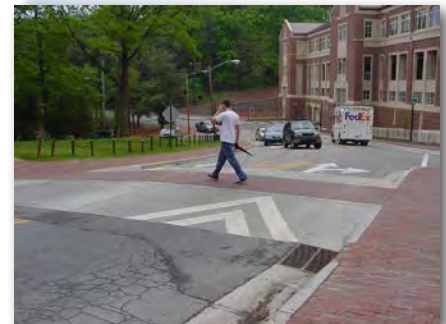
Raised crosswalk: University of North Carolina, Chapel Hill, NC (Credit: Ryan Snyder)
