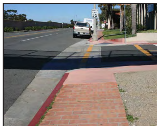
Brick sidewalk paving on South El Camino Real
