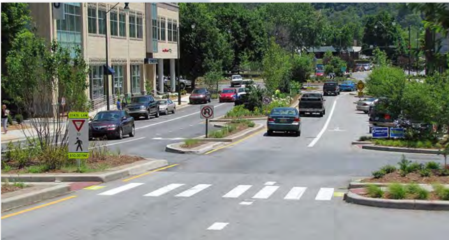
Curb extensions and medians make crossing multi-lane streets safer and more manageable (Credit: Dan Burden)
