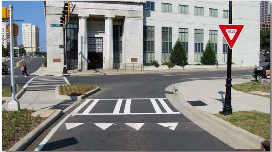
Multiple tools can be employed to improve uncontrolled crossings (Credit: Dan Burden)
