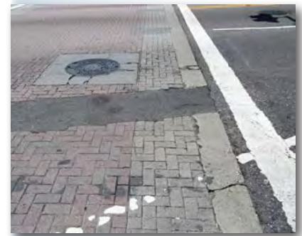
Decorative crosswalk treatments made of distinctive materials can become uneven over time (Credit: Ryan Snyder)
