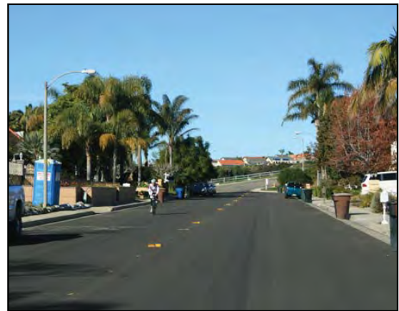
Sidewalk with driveways
