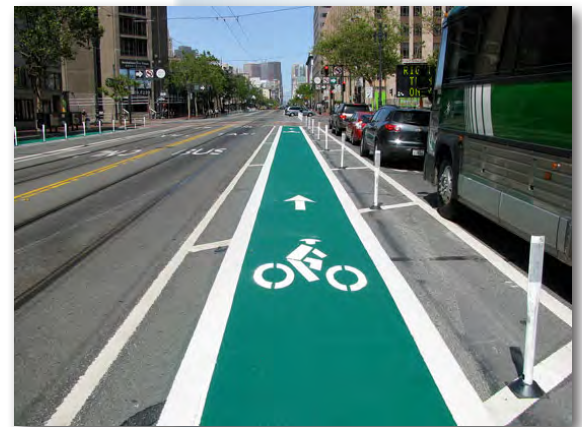
Colored and buffered bicycle lanes: San Francisco, CA (Credit: San Francisco MTA)
