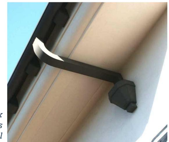
*Example. Copper leader box used when downspout is against the wall*
