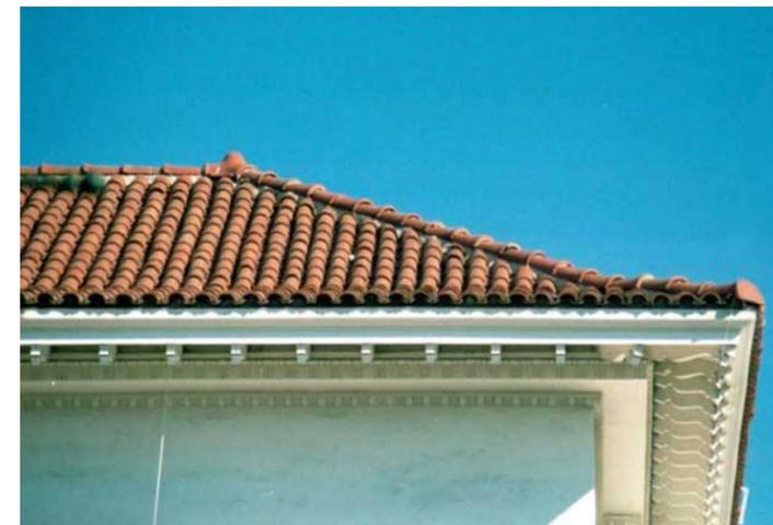
*Example. Hip tiles capped and packed with mortar*
