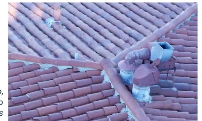
*Example. No hip cap, ridge tiles shall lap over hip tiles*
