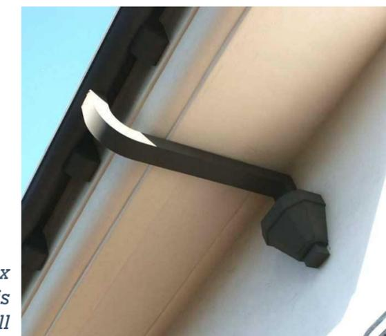
*Example. Copper leader box used when downspout is against the wall*
