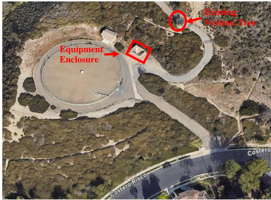
Figure 1 – Existing Site Conditions
