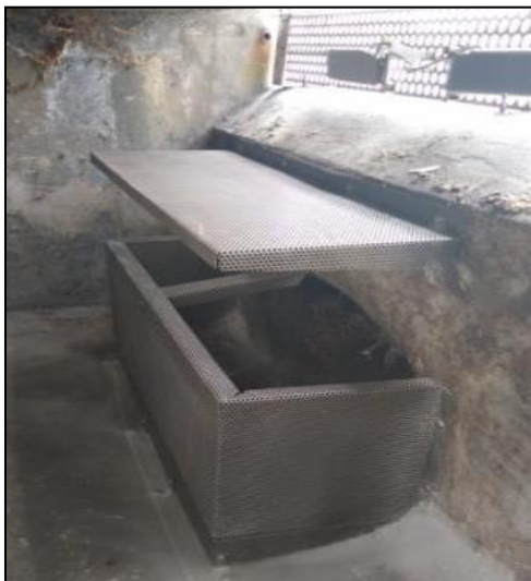
Full-capture Connector Pipe Screen (CPS):
