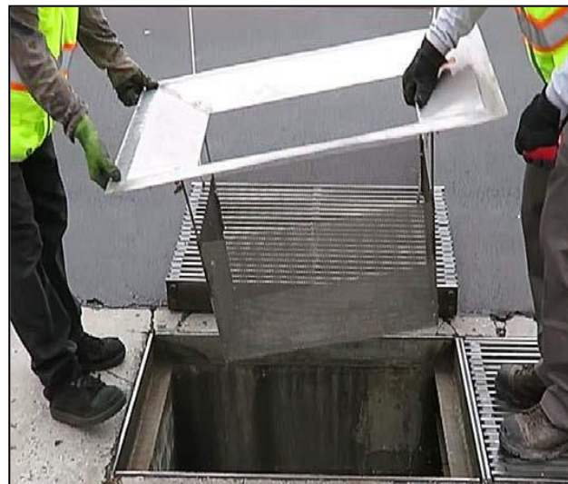
Full-capture Grate Inlet Trash Screen (GITS):
