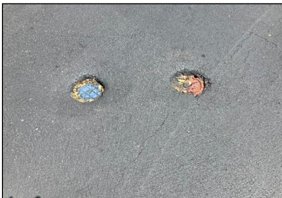
Existing Water Valve Cans
