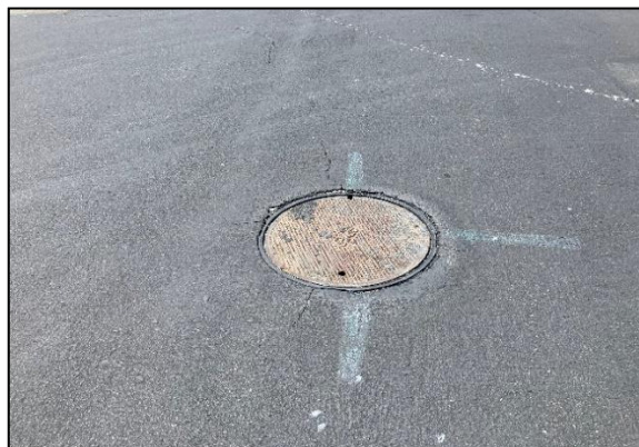
Existing Sewer Manhole
