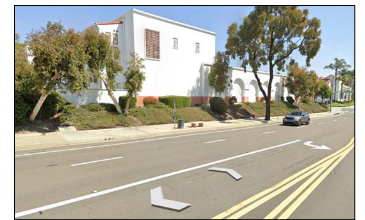
(F) VIEW FROM SOUTHWEST SIDE SCALE: N.T.S.
