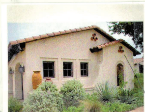
FALSE CLAY PIPE VENT
