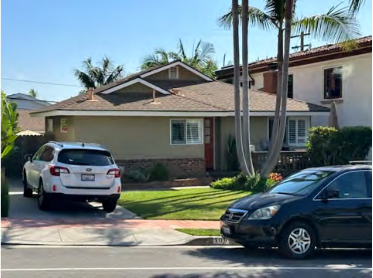
109 W Paseo de Cristobal Semi-modernized beach cottage structure
