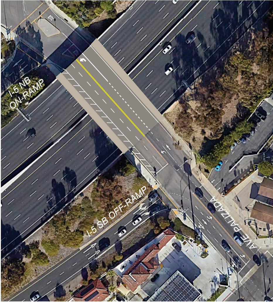
EXISTING CONDITION ON AVE PALIZADA BETWEEN I-5 NB ON-RAMP AND SB OFF-RAMP
