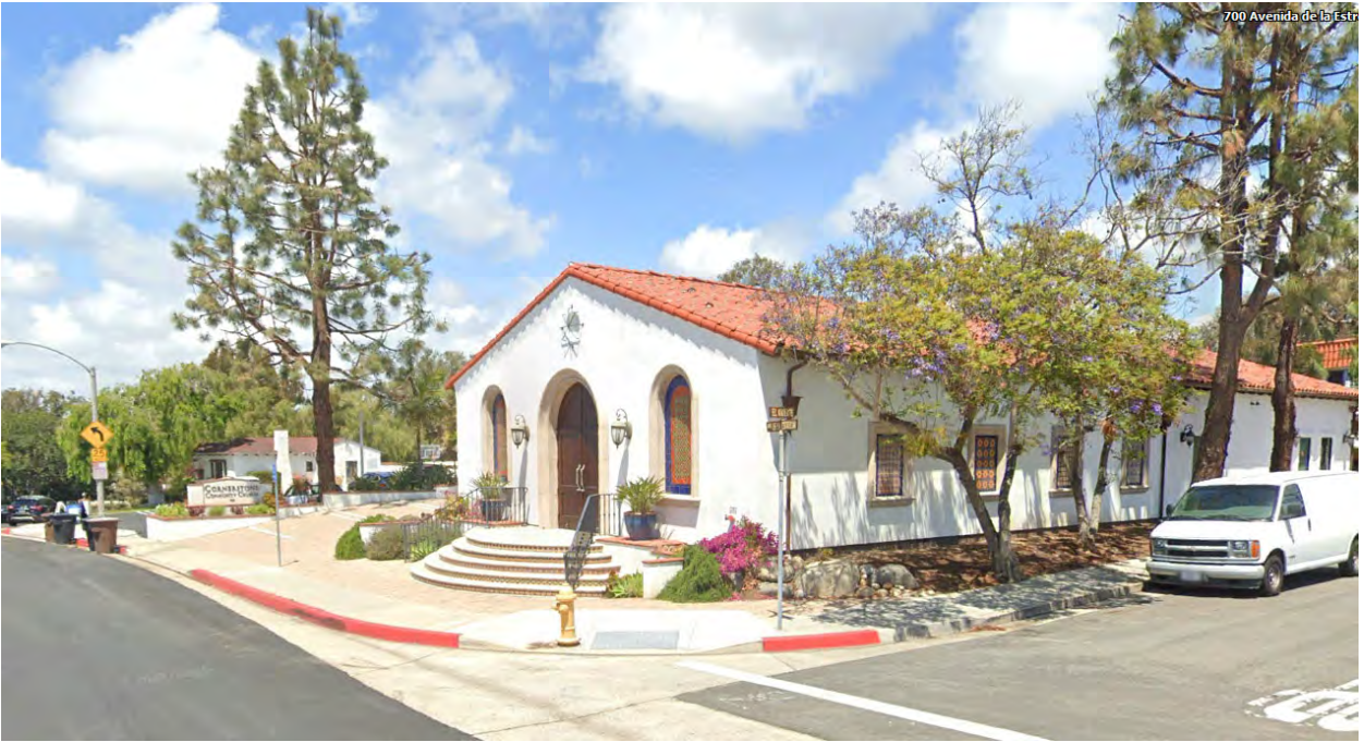
Photo 1: View Looking North from Avenida De La Estrella at the Existing Church
