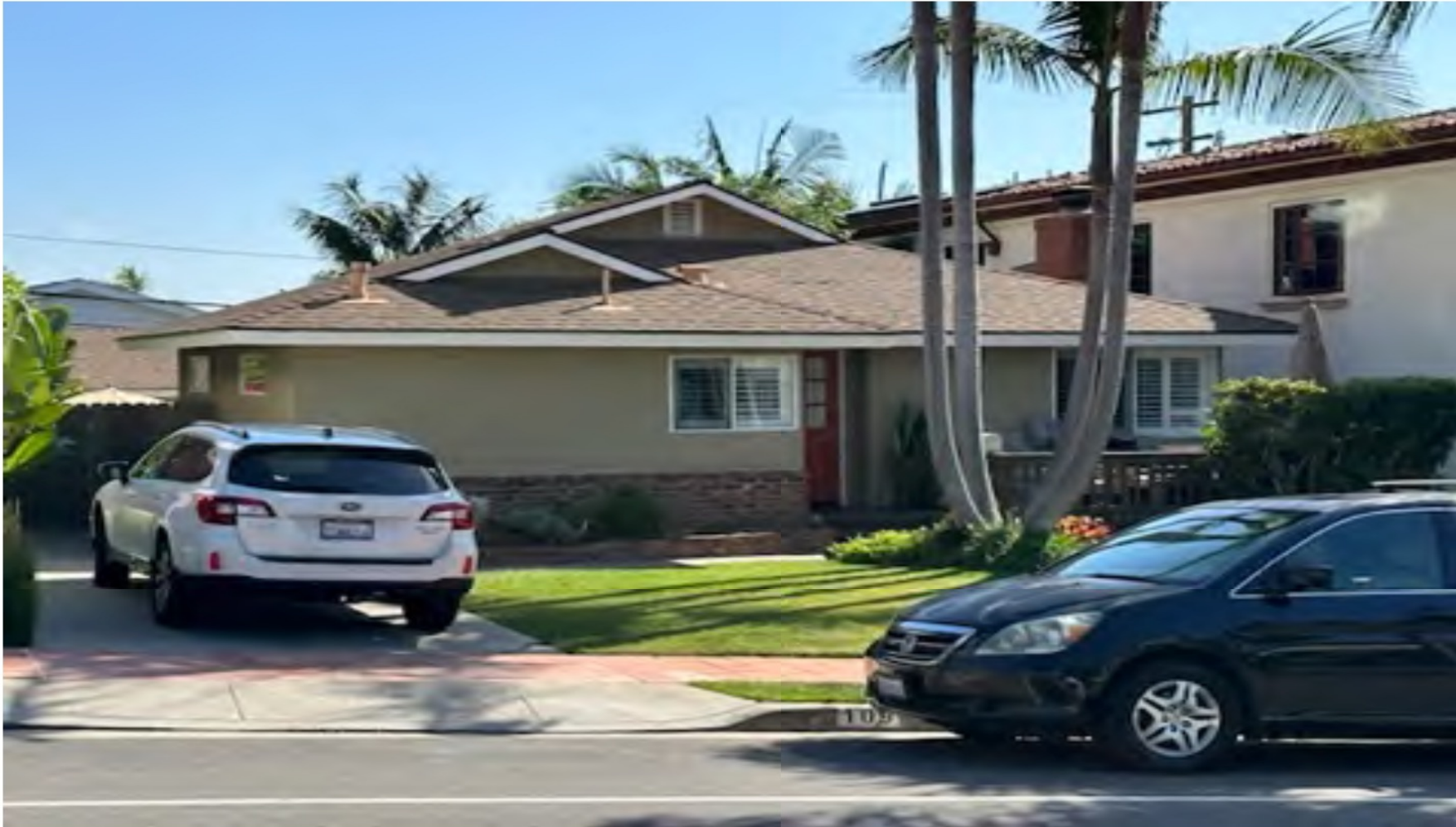
109 W Paseo de Cristobal Semi-modernized beach cottage structure
