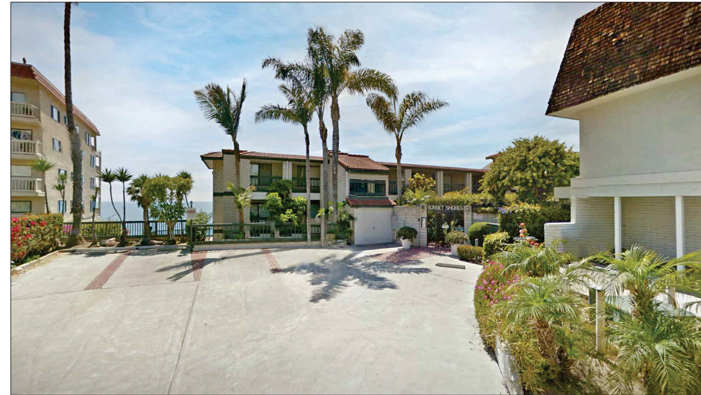
VIEW FROM CORTO LANE BEFORE
