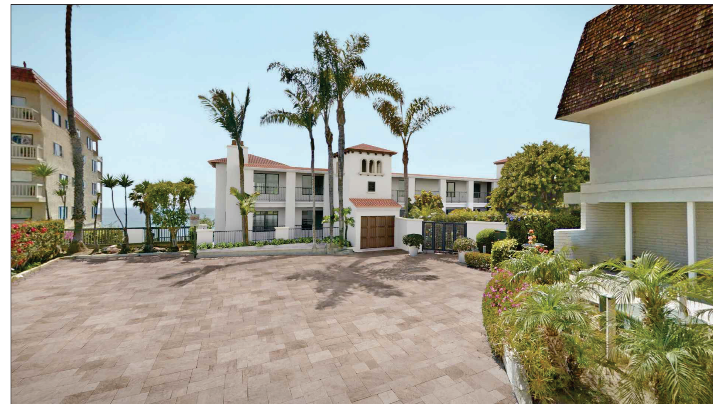
VIEW FROM CORTO LANE AFTER
