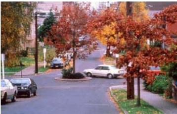
Traffic circles are a raised island located in the center of an unsignalized intersection. Drivers must maneuver around the central island rather than proceeding straight. Traffic circles replace two and four way stop controls on local streets.
