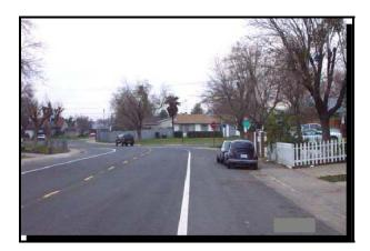
Lane striping can be used to create formal bicycle lanes, parking lanes, or edge lines. As a neighborhood traffic management measure, they are used to narrow the travel lanes for vehicles, thereby inducing drivers to lower their speeds.
