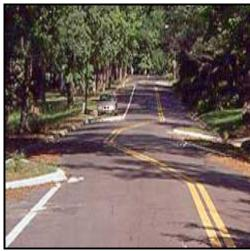
An Angled slow point is a variant of a chicane or one-lane choker. An angled deviation to deter the path of travel so that the street is not a straight line (by the installation of offset curb extensions).
