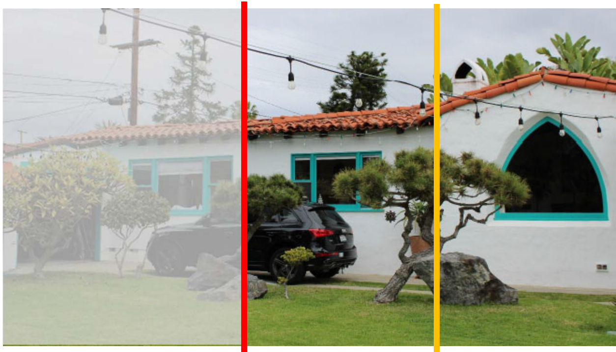
Image 1 – Portion of the existing West Elevation
