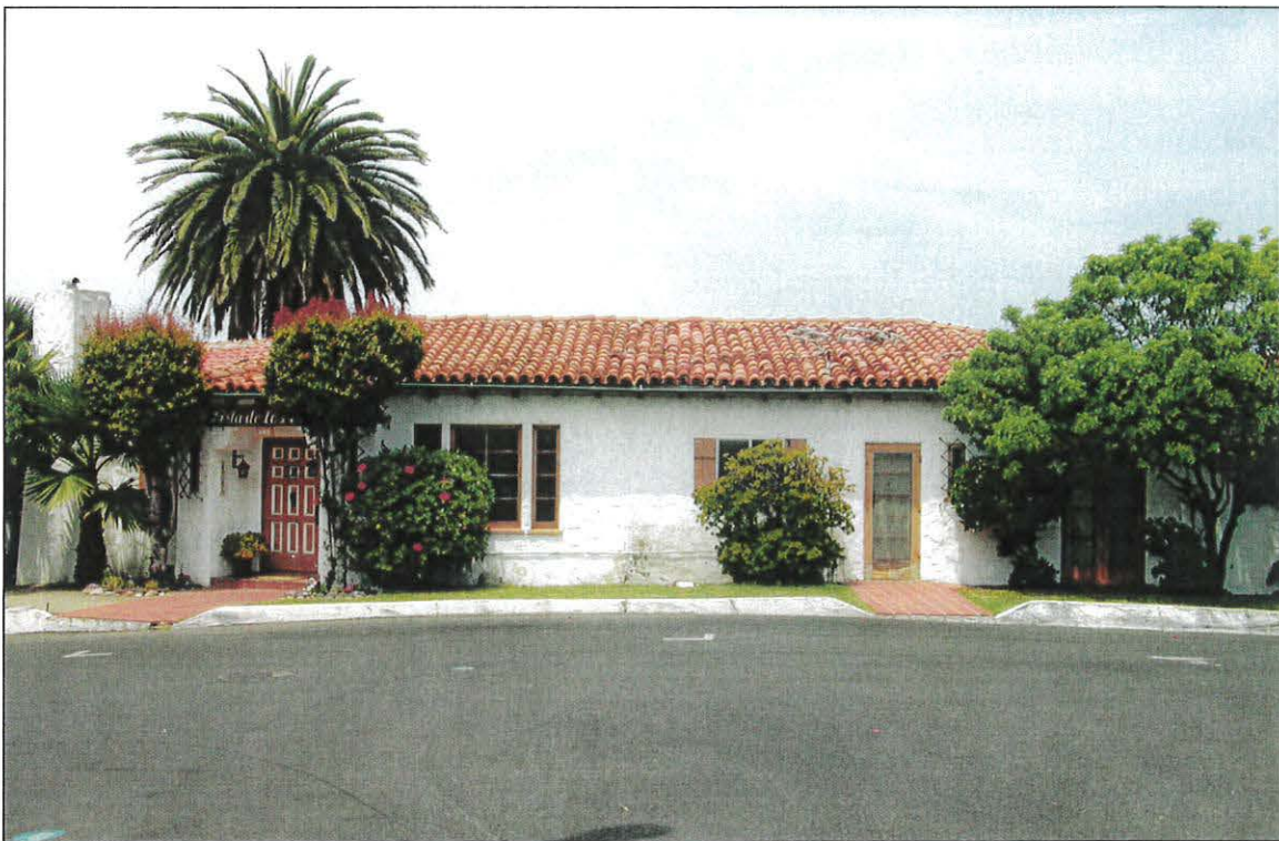
Photograph 6: Existing residence, east elevation, view west, 2002 (Chattel Architecture, CA)
