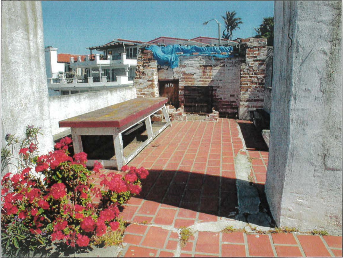
Photograph 17: South garden, terrace walls, trellis and barbecue, view northeast, 2002 (CA)
