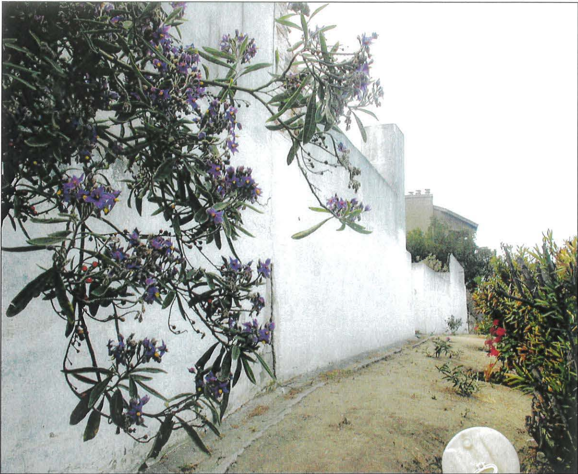
Photograph 11: Subject property, west retaining wall, view south, 2002 (CA)
