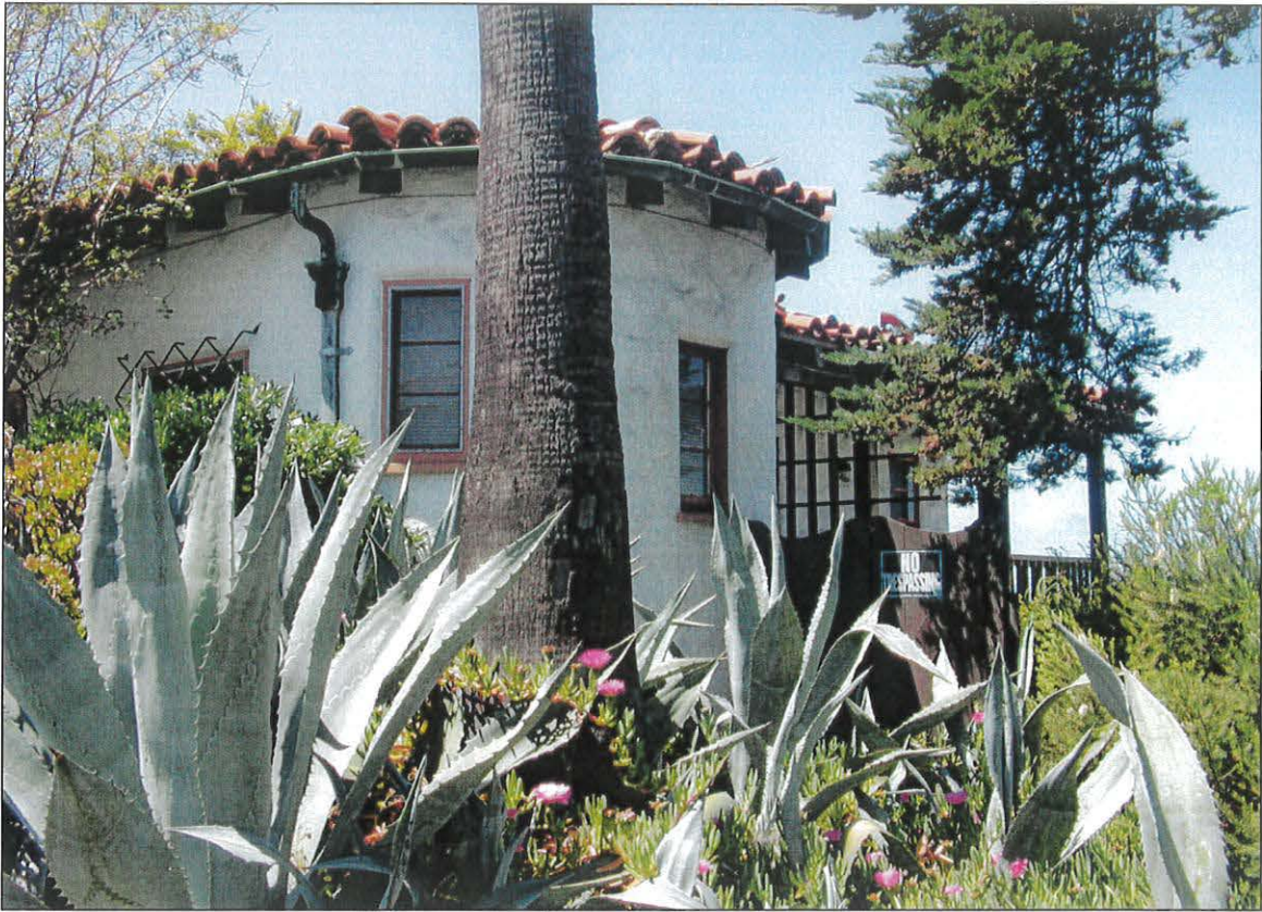
Photograph 7: Existing residence, east (left) and north (right) elevation, view southwest, 2002 (CA)
