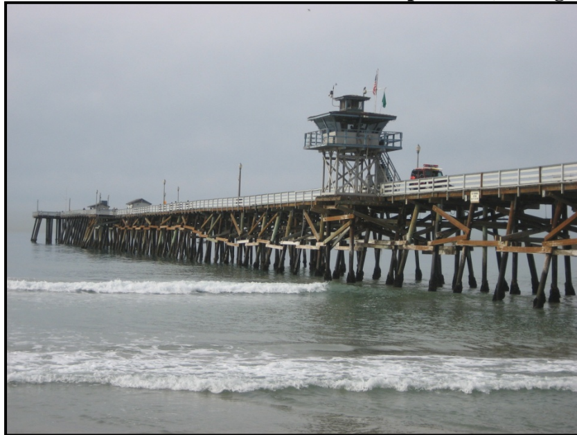
Figure 4-11 Overview of San Clemente Municipal Pier (looking west)
