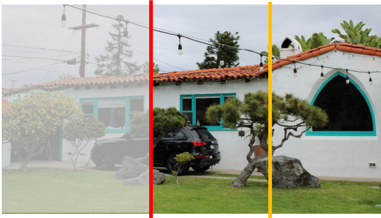
Image 1 – Portion of the existing West Elevation
