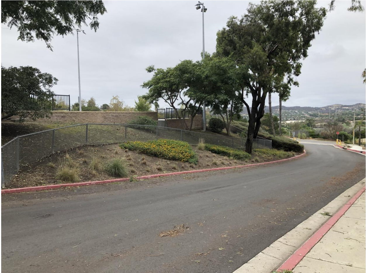
Figure 4.3-2 SLOPE LANDSCAPING WEST SIDE OF PARK ENTRY DRIVE; VIEW TO THE NORTHEAST
