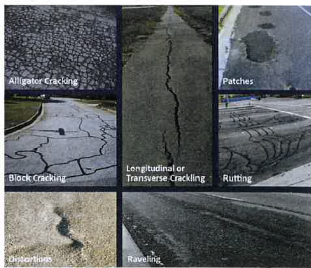
Figure 2 – Pavement Distortions
