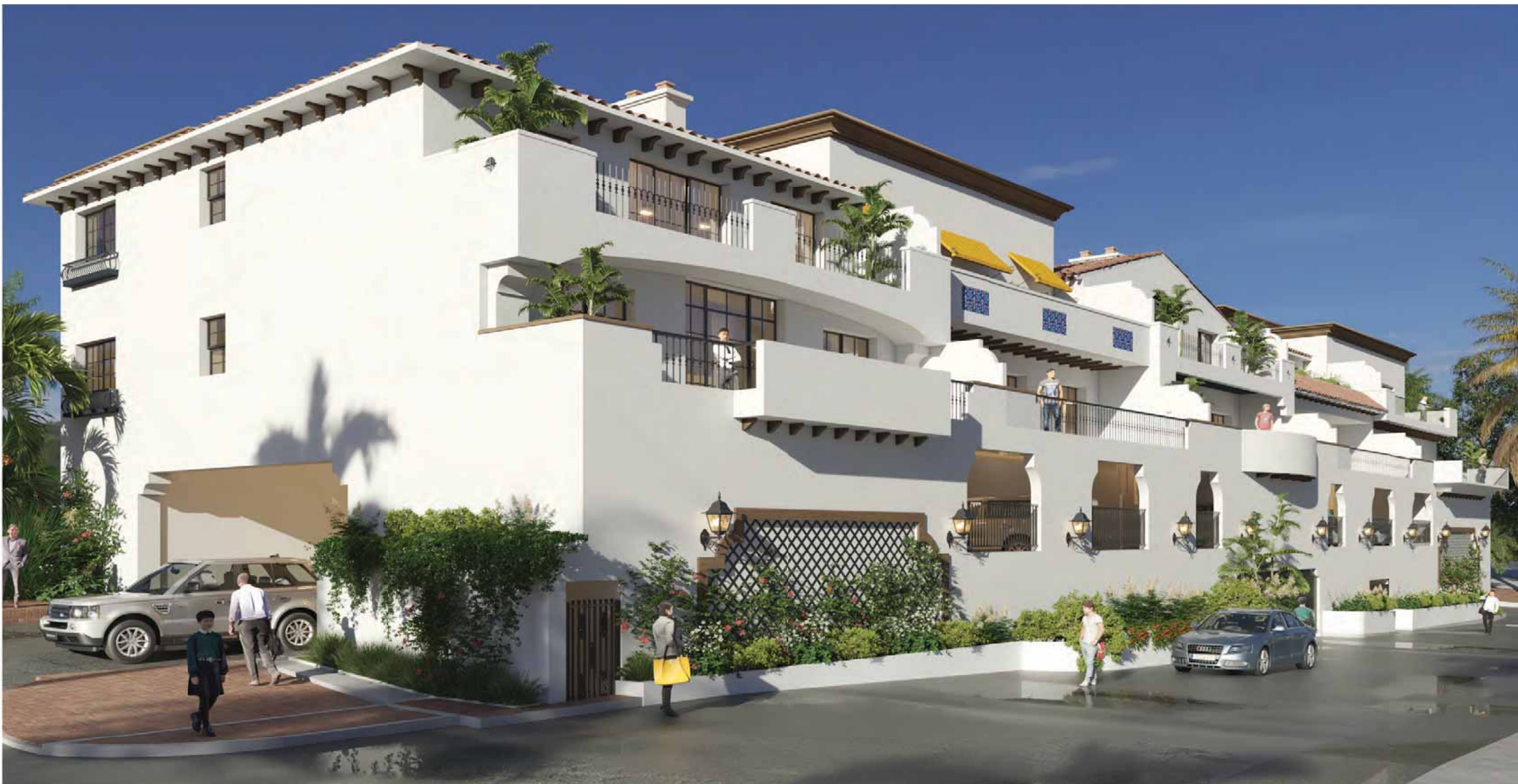
FROM ALLEY LOOKING NORTHWEST
