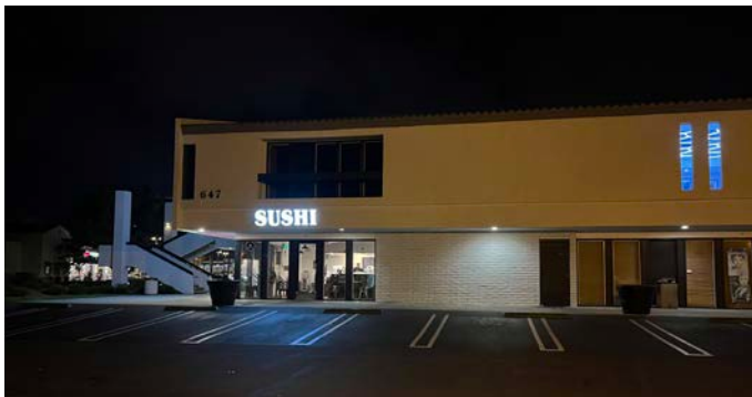
Photo 15: Signage and building security lighting (≈3-20 fc)
