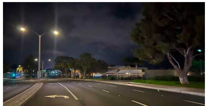
Photo 8: Street lighting near project site ( \approx 2-3 fc)
