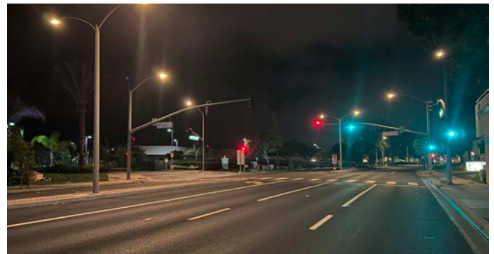
Photo 10: North on Camino de los Mares near Sr. Housing ( \approx 2-3 fc)
