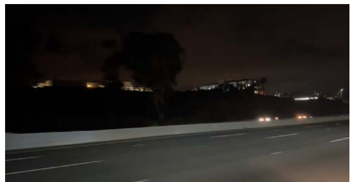
Photo 6: Southbound Freeway of existing site (≈1 to 2 fc)
