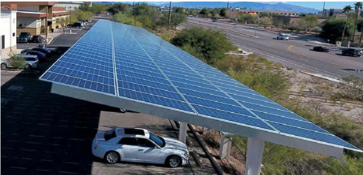
Solar carports being considered with a single post cantilever design
