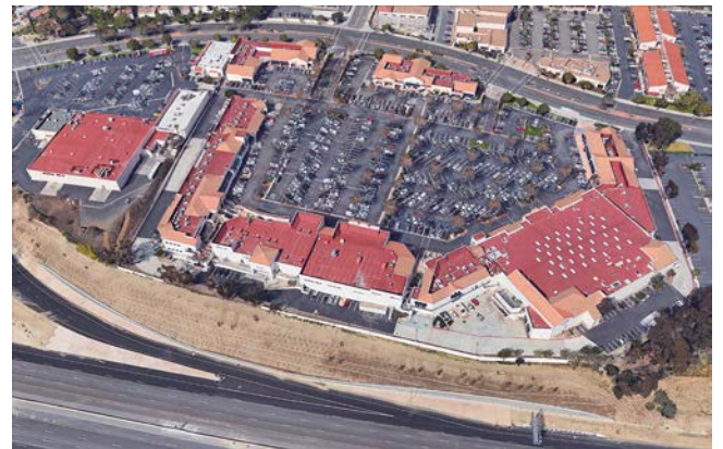
Visual Assessment Unit 2: Commercial Retail
