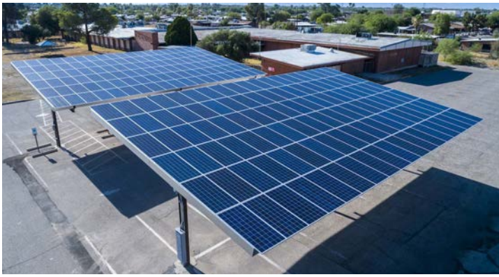
Solar carports being considered with a single post cantilever design
