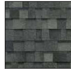
EXAMPLE OF ROOFING COLOR
