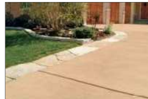
EXAMPLE OF POURED IN PLACE CONCRETE PIECES
