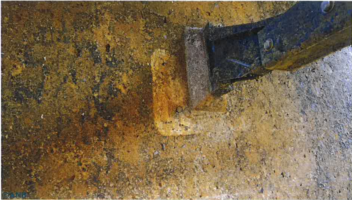
Figure 5: Abandoned steel bolts on walls throughout
