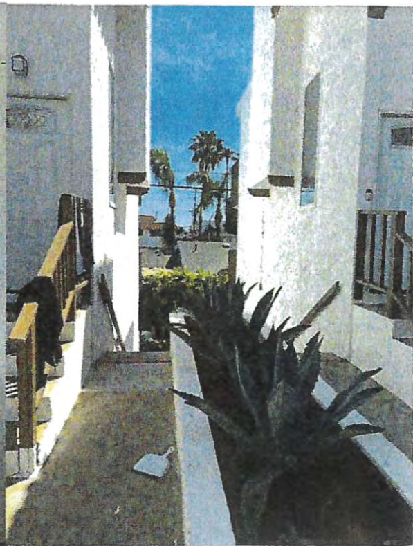
walkway to unit C below
