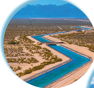
Colorado River Aqueduct
