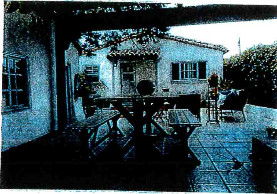
View from South Wall to rear of home
