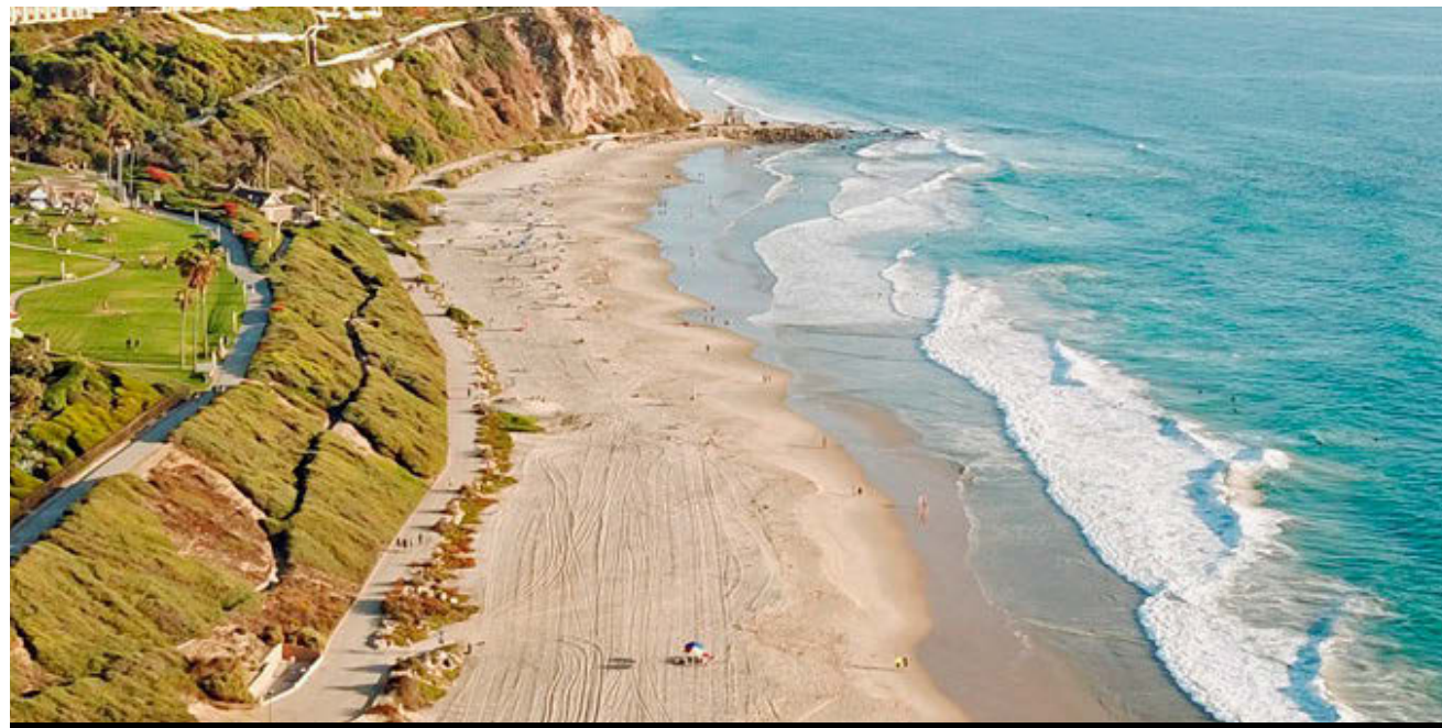
Native Planting For Slope Stabilization
