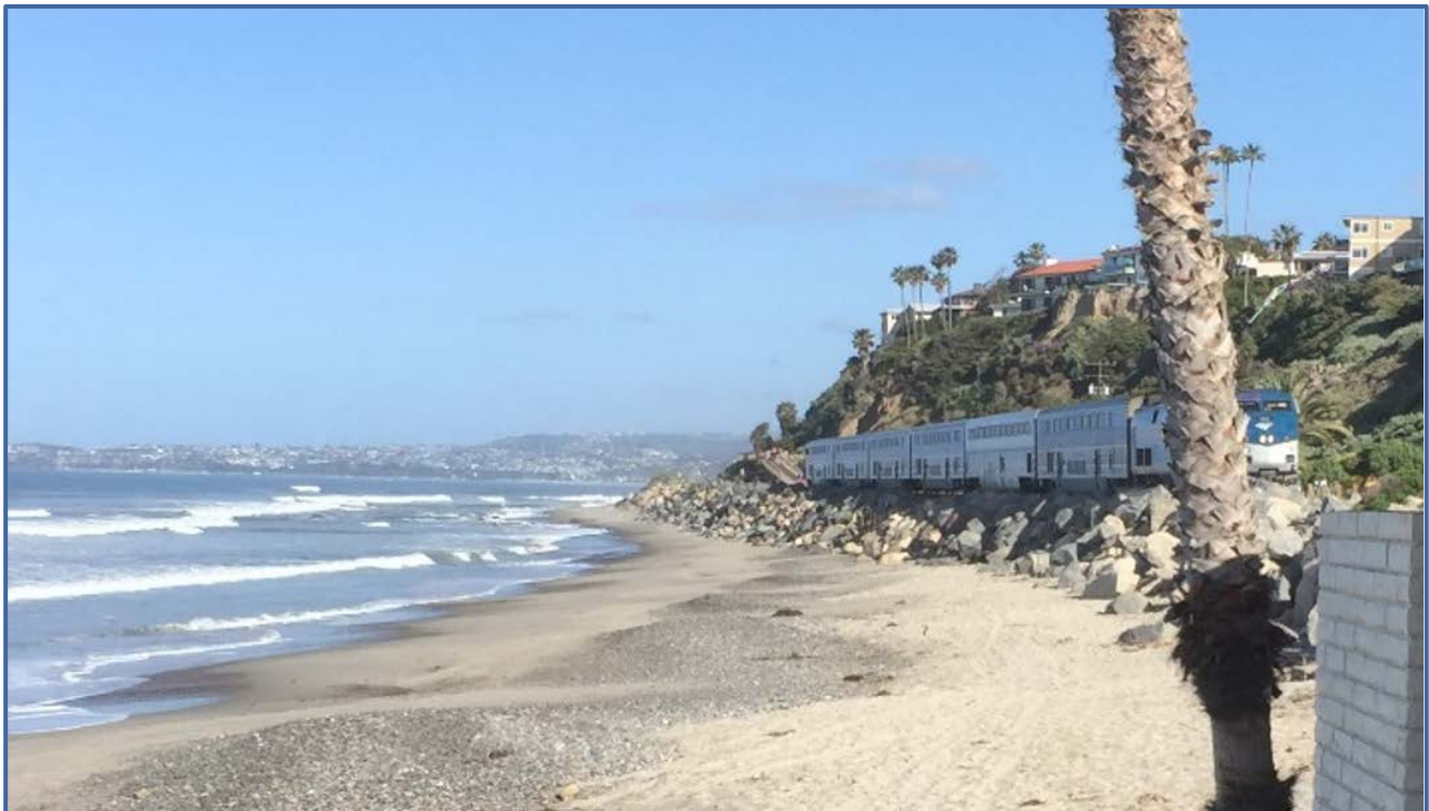
Figure 4-3. Existing Railroad and Revetment in San Clemente
