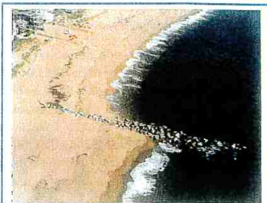
Figure 7-2. Cross-Shore Rock Revetment
