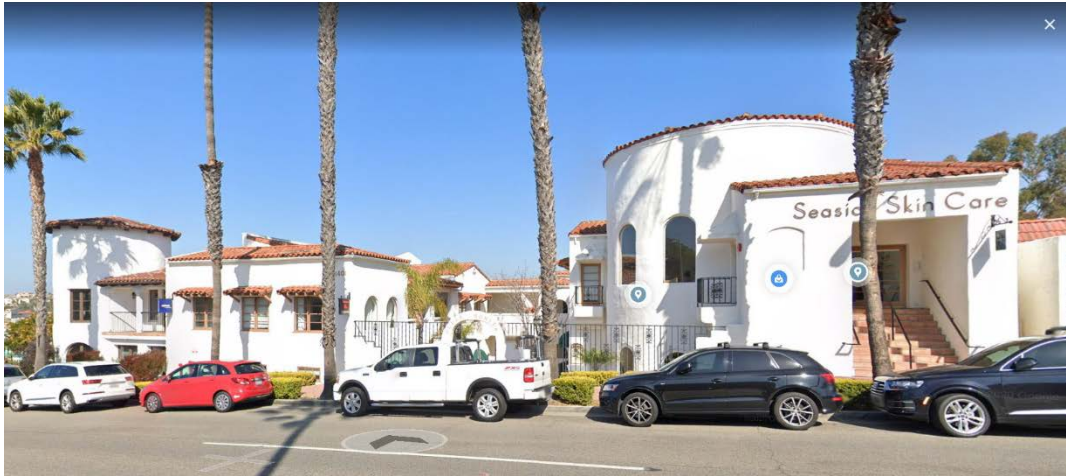
Figure 2 – Existing Office Location
