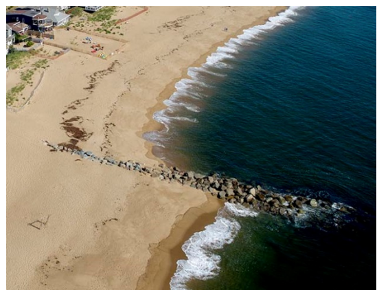
Figure 7-2. Cross-Shore Rock Revetment
