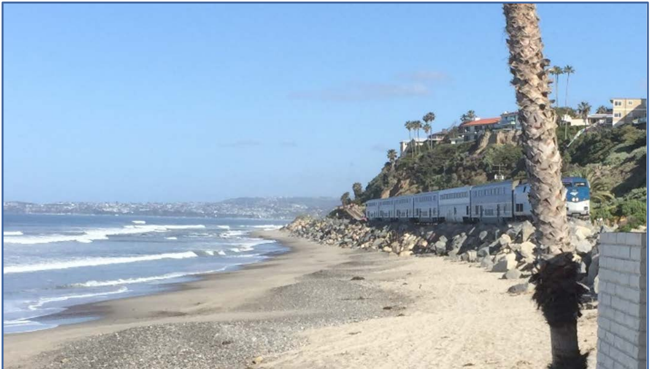
Figure 4-3. Existing Railroad and Revetment in San Clemente
