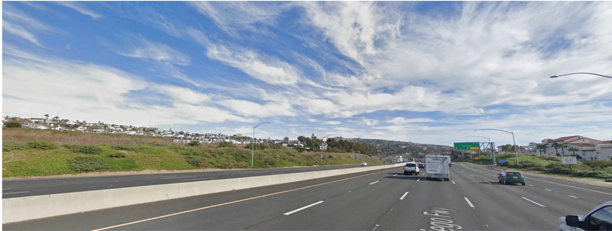
SAN DIEGO 5 FREEWAY(SOUTH) (EXISTING)
