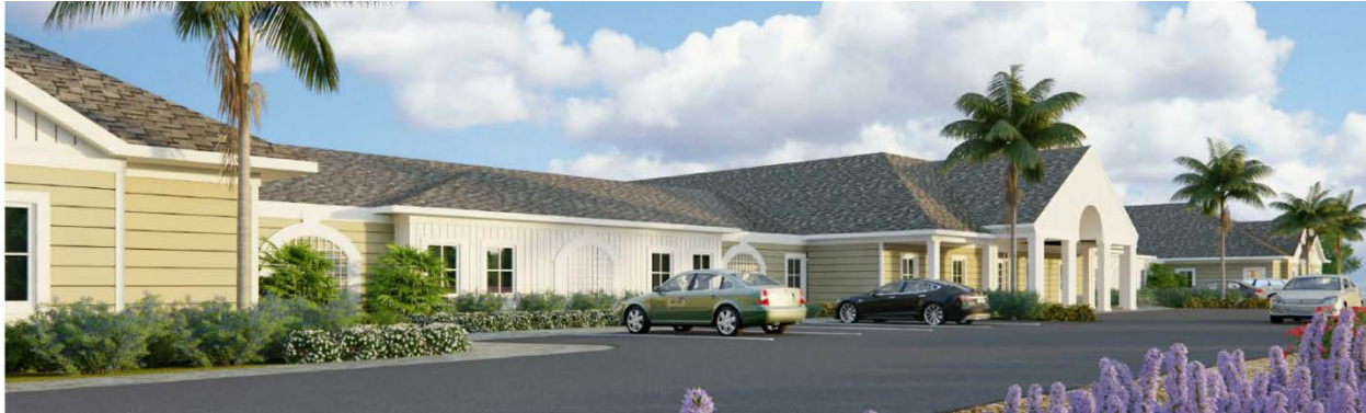
Figure 3 – Main Building Entrance
