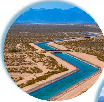
Colorado River Aqueduct
