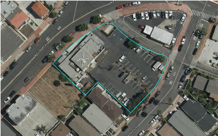
Figure 1 – Existing Site Conditions
