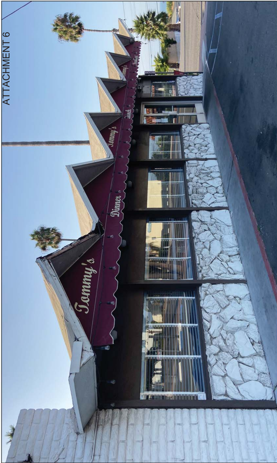
Plate 10 View of the West Façade of the Building Showing the 1975 Faux Fieldstone Veneer and Folded Plate-Style Roof, Facing Southeast
