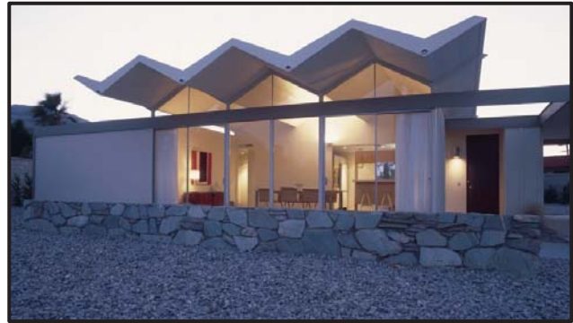
Plate 26: Wexler's 1962 Steel Development House #1 in Palm Springs. (Photograph courtesy of David Glomb)
