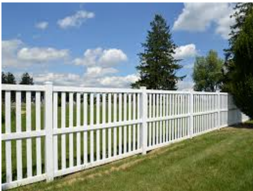
Below is a non-compliant barrier fence. The horizontal members must be 45 inches apart to prevent a climbable condition.
