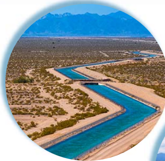
Colorado River Aqueduct
