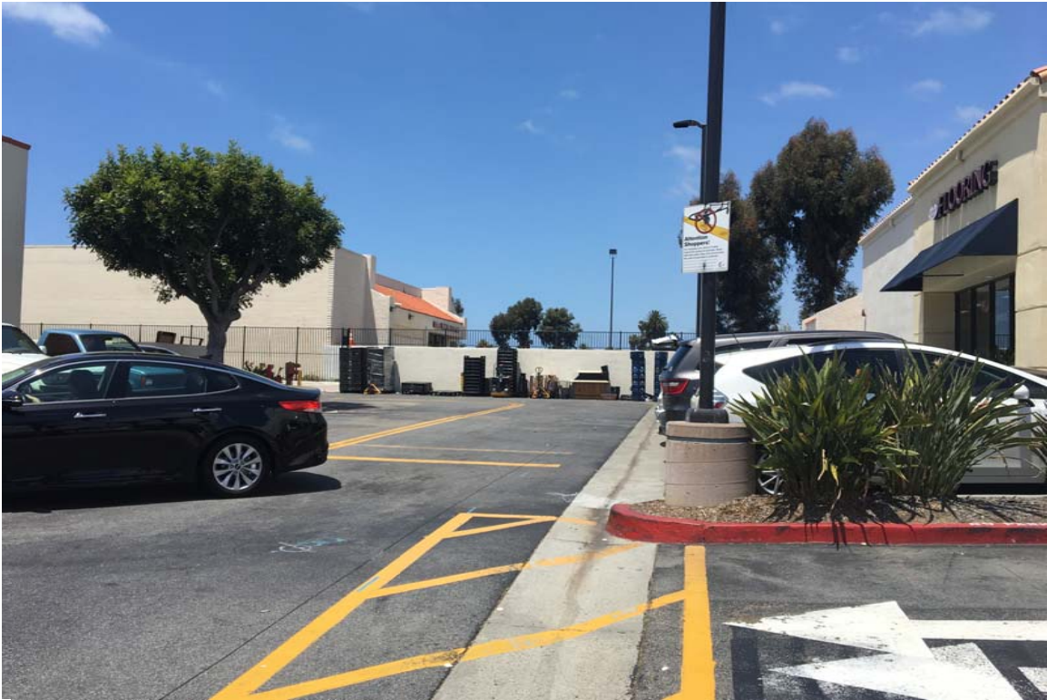
Wall between plazas (existing)
