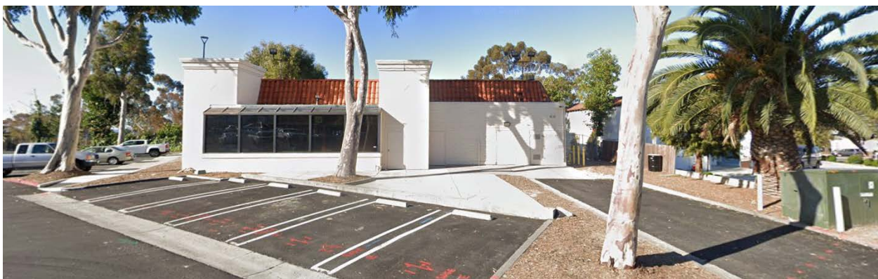
Figure 1: Outparcel Building (610) Proposed to be Demolished
