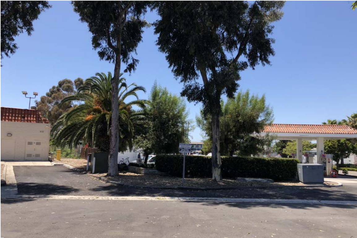
Outparcel building (existing)
