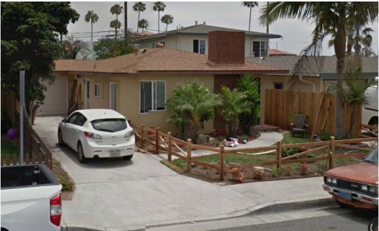
Figure 1 – Existing Site Conditions
