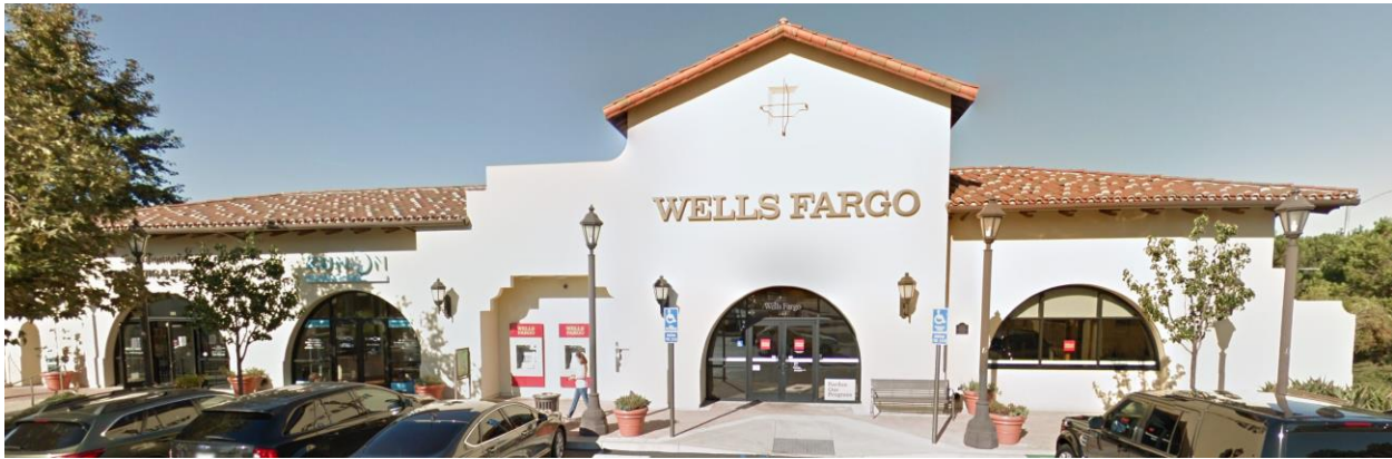
Figure 5: Arched Glass Matching Entry Inset
