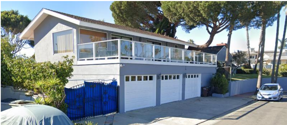
Figure 1 – Existing Site Conditions
