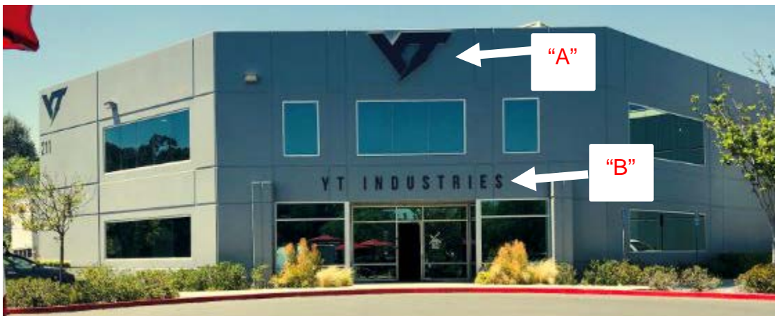
Figure 1 – Interior Facing Walls Signs "A" and "B"
