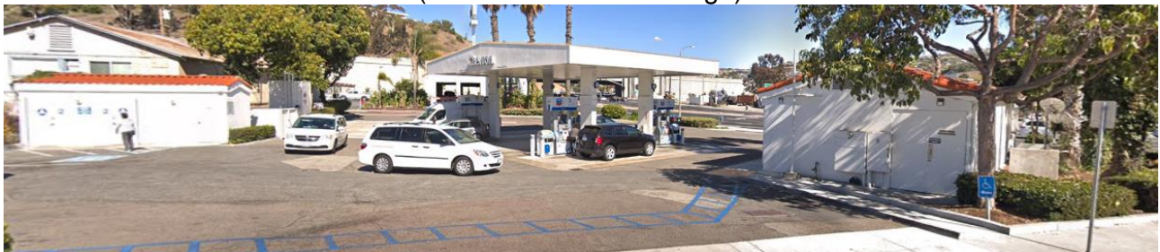
Figure 1b: Existing Conditions (Calle Industrias Frontage)
