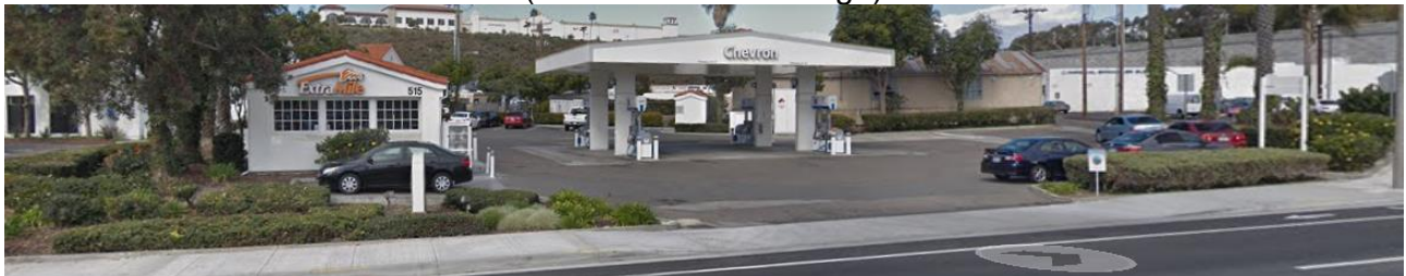
Figure 1a: Existing Conditions (Avenida Pico Frontage)
