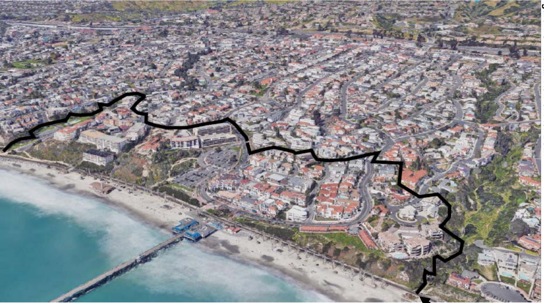
Figure 1-3 – Aerial View of Pier Bowl
