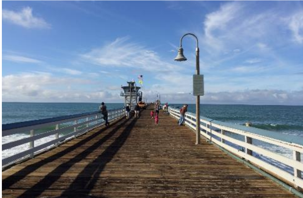
San Clemente Pier
