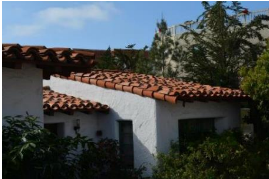
Two-piece Spanish tile with random mortar packing and booster tiles
