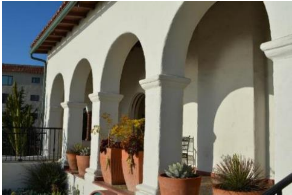
Arcade on rear facade of Casa Romantica
