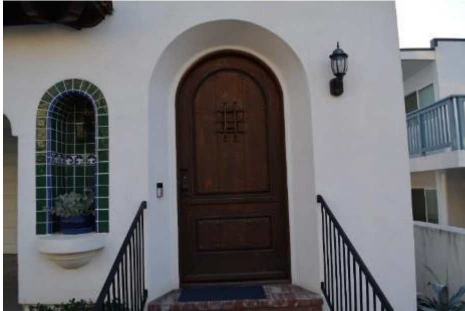
Entrance with inset wood door
