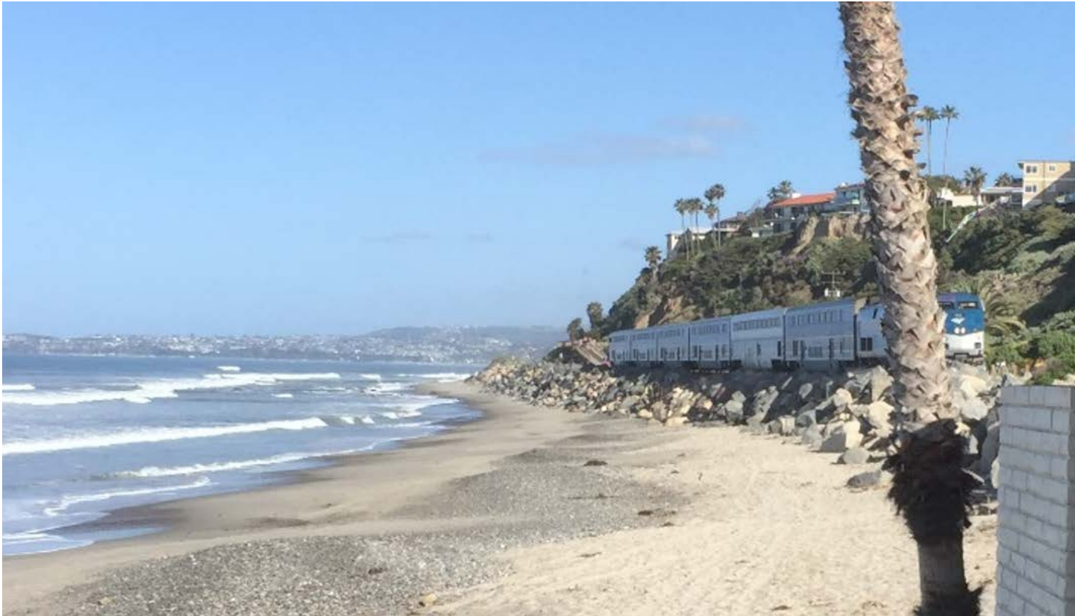
Figure 4: Existing LOSSAN Railroad Corridor, North Reach, San Clemente
