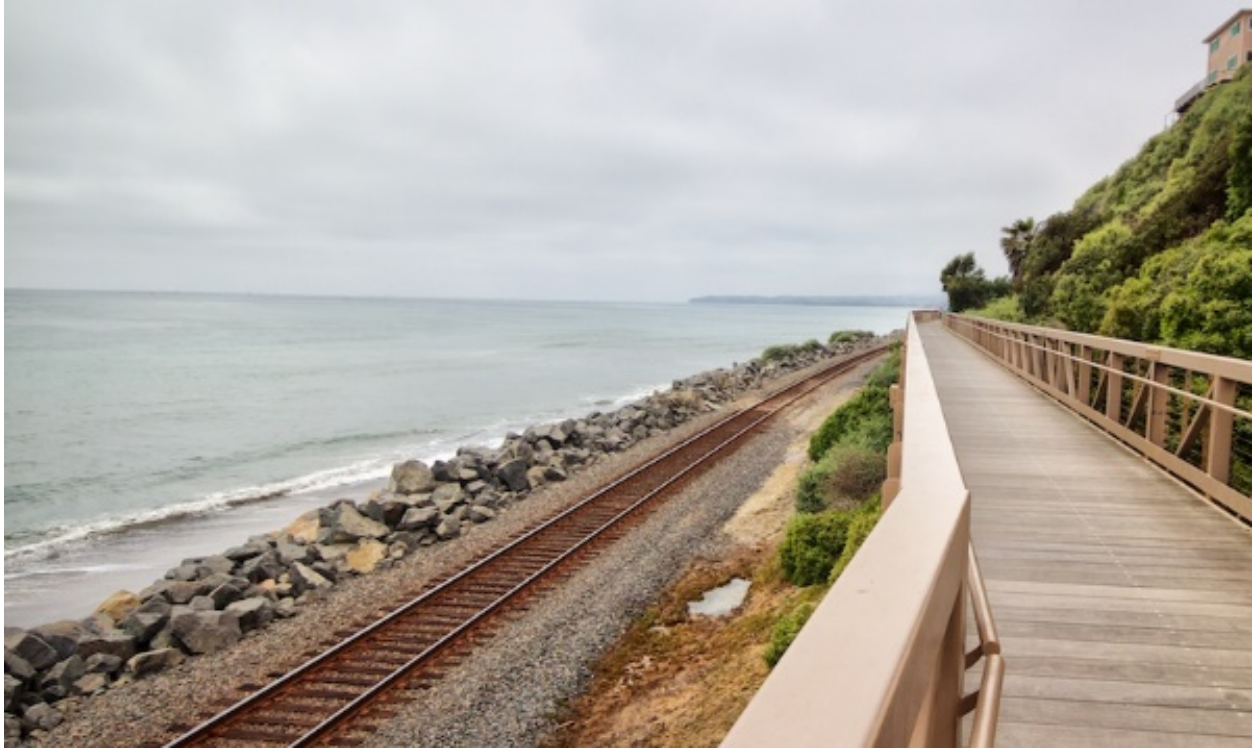
Figure 32: Coastal Squeeze at Mariposa Point
