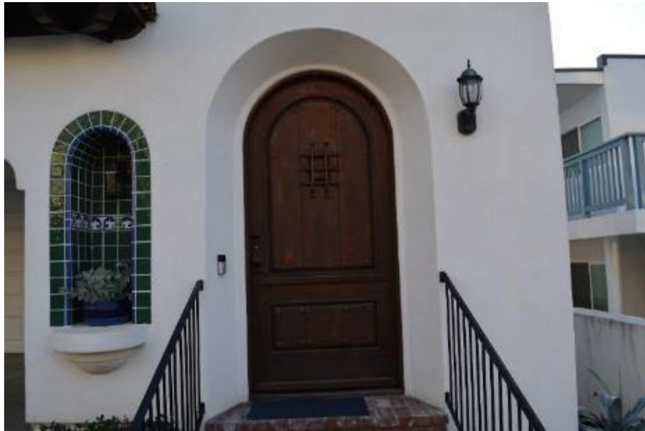
Entrance with inset wood door
