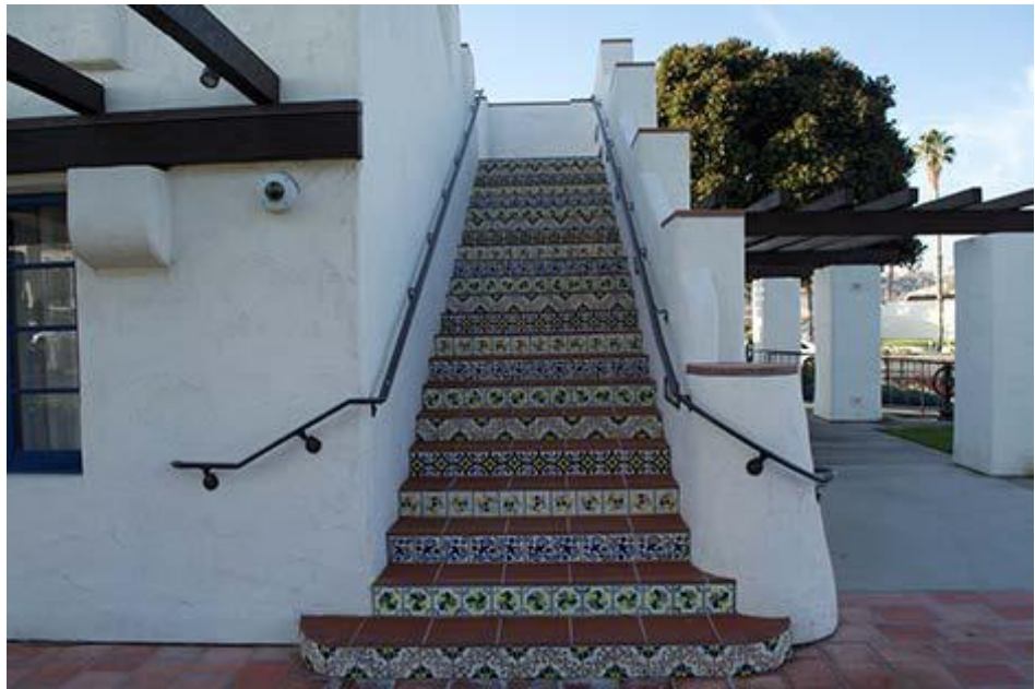
Tile risers on exterior stairway of beach club in North Beach
