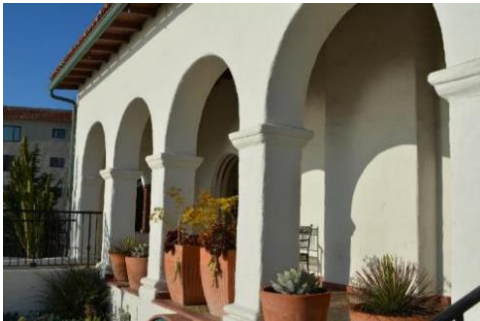
Arcade on rear facade of Casa Romantica
