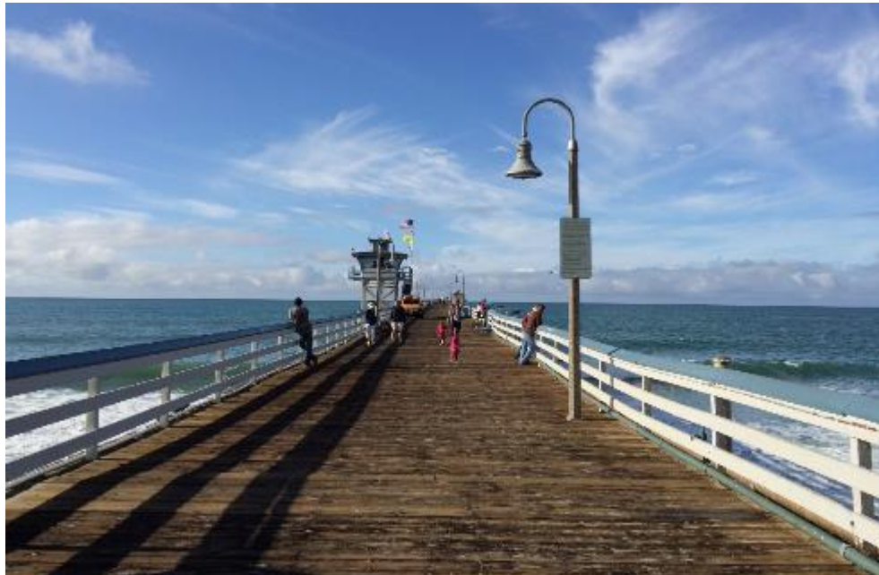
San Clemente Pier
