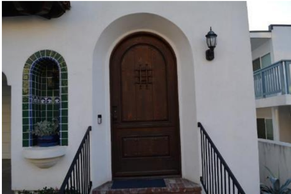
Entrance with inset wood door
