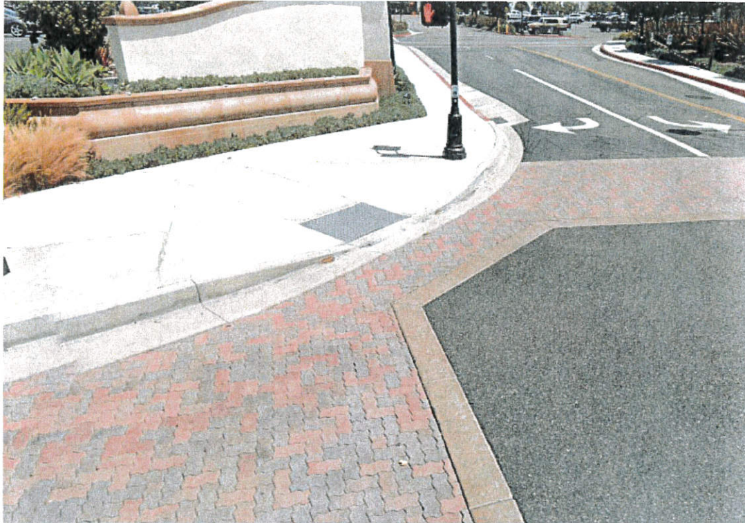
Photo 3. Example of existing City standard decorative paver in crosswalk on West Avenida Vista Hermosa.
