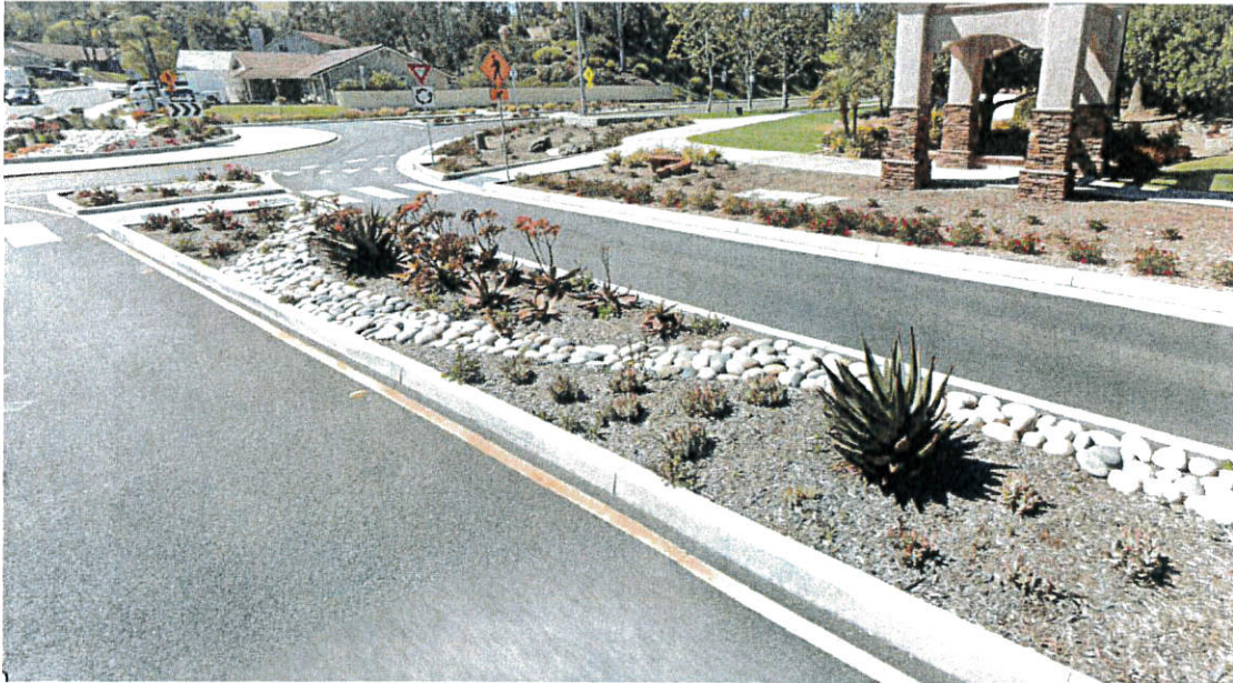
Photo 7. Example of meandering cobble stone and decorative mulch (at Camino Del Rio and Camino De Los Mares roundabout).
