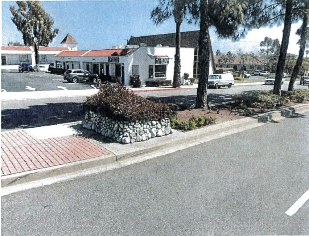
Photo 5. Existing cobble planter box to be removed (on Camino De Estrella west of Mira Costa). Red stamped concrete and grey concrete median border to be removed.
