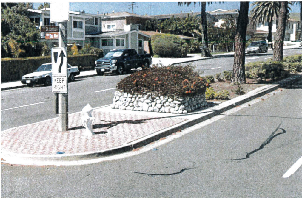
Photo 6. Existing cobble planter box to be removed (on Camino De Estrella east of Vista Del Mar). Red stamped concrete and grey concrete median border to be removed.
