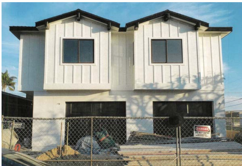
Figure 1: Existing Site Conditions
